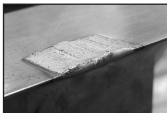
Repaired part ready for grinding.
